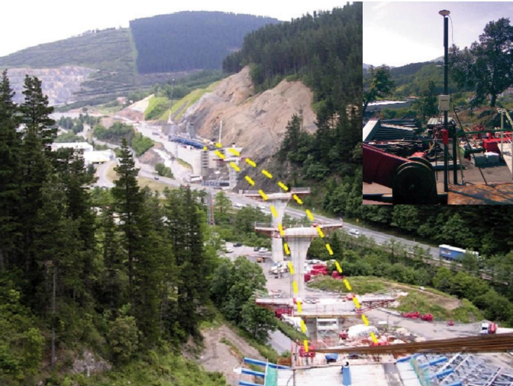
**Arbizelay's bridge, 380 meters long, 6 spans high, 5 pylons and 12 meters wide is part of the AP-1 Vitoria - San Sebastián Motorway and is located near the city of Mondragon. Thanks to Leica GNSS technology, it was possible to successfully complete the manoeuvre of incremental launching of the bridge's deck over the pylons with an error of less than 3 centimetres.**
