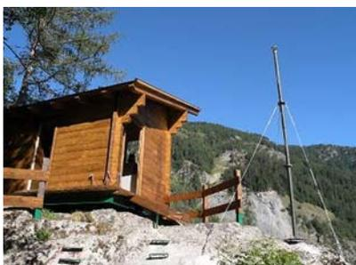
of the buffer battery on site. The power system consists of solar panels and a methanol tank system. A special electronic device controls automatically and intelligently the correct power input to the monitoring equipment between the solar panel and the methanol tank system.
