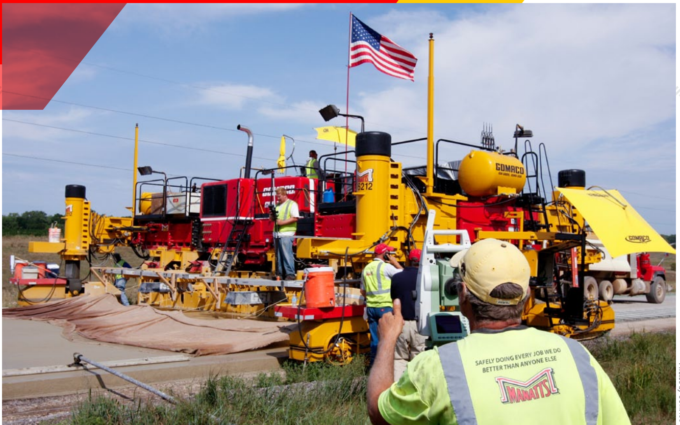
A technician uses a Leica robotic total station to check elevation of the new concrete slab.
