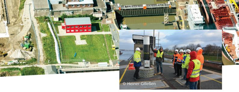
After collecting and analysing new and previous data for three months, the building of the chamber could start. During construction, the chamber walls next to the building site will be continuously monitored three times per hour for any standard deviations (2 mm) and for any deformation activity of more than 15 mm from the position and height of each measured point being monitored.
