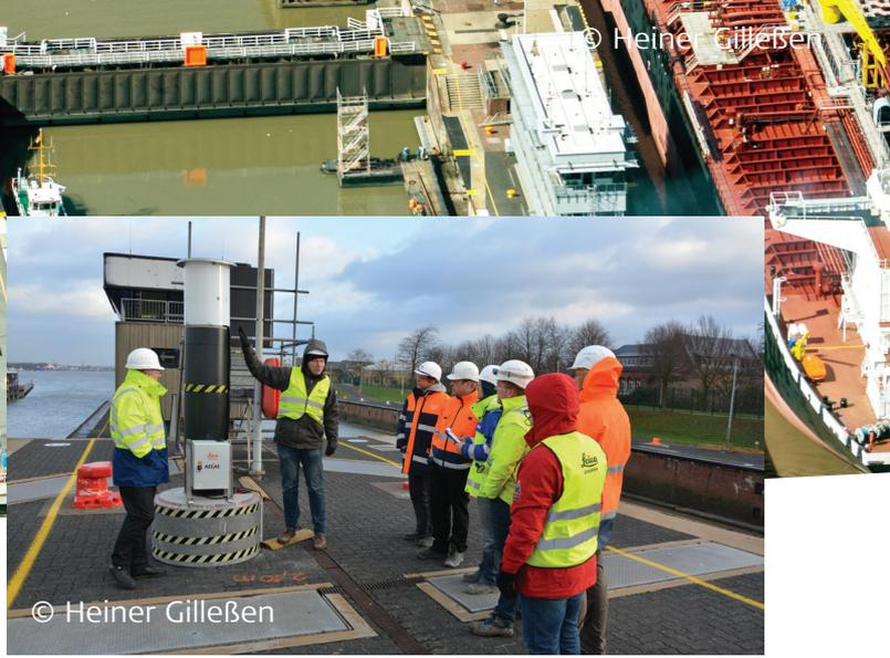
After collecting and analysing new and previous data for three months, the building of the chamber could start. During construction, the chamber walls next to the building site will be continuously monitored three times per hour for any standard deviations (2 mm) and for any deformation activity of more than 15 mm from the position and height of each measured point being monitored.
