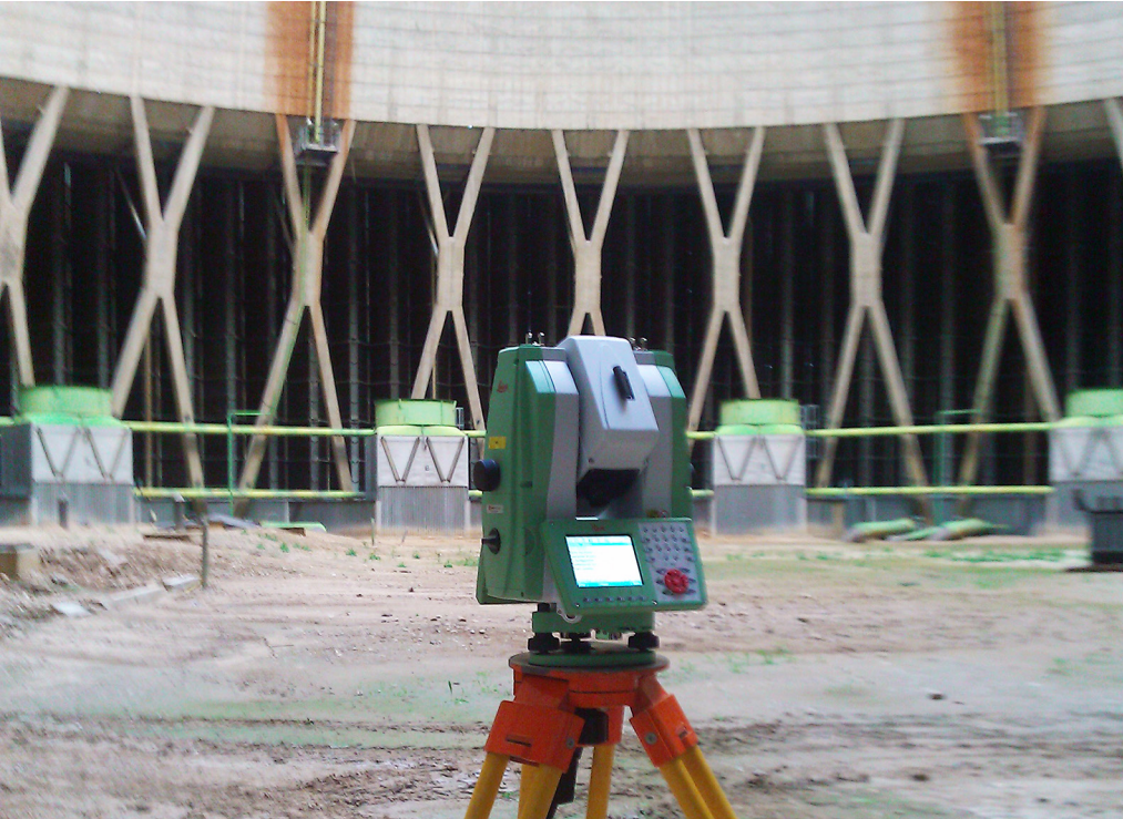
The Leica Nova MS50 scanning the inner shell of one of the cooling towers.
