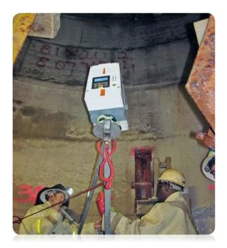
cessing point cloud data and 3D Reshaper for modeling. Owing to difficulties with the fine tolerances between the extent of the infrastructure and the tunnel design, 3D MSI surveyed down to -3,900m (2.42 mi) to provide a comprehensive analysis of problem areas prior to the installations. A total of 240 separate scans were taken for all 3 of the declines, equating to a combined distance of 3.5 km (2.2 mi).
