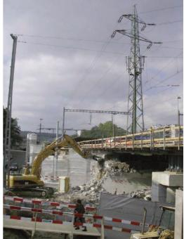
During demolition of parts of the foundation of the power line pylon, the monitoring systemwas used to detect 3D deformations and the resulting change in tilt.
