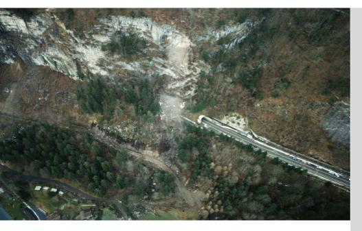
In January 2003 there was a fall of approximately 150 m<sup>3</sup> of rock from above the Chüebalm tunnel in Iseltwald/Interlaken. The falling rock punctured the tunnel near the western entrance and blocked the highway.
