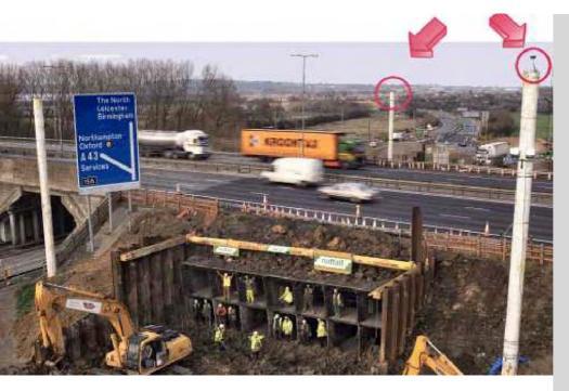
In 2002, Edmund Nuttall won the contract to improve the interchange of the M1 motorway and the A43 trunk road at junction 15a in Northamptonshire. The primary element of the project comprised a boxjack through the current motorway embankment, in order to upgrade the existing A43, running beneath the M1, to dual-carriageway status.
