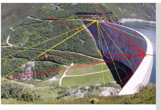
The Gotthard base tunnel will be the longest rail tunnel in the world upon its completion. There is a small risk that construction of the tunnel will cause movements in the land above because of water being drained from the rock mass. Above the area of the tunnel are three of the largest dams in Switzerland.
