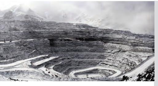
Since 2003 the Kumtor gold mine has been using Leica GeoMoS as their main automatic deformation monitoring system. Periodic manual monitoring and geotechnical instrumentation are still in use for added safety.
