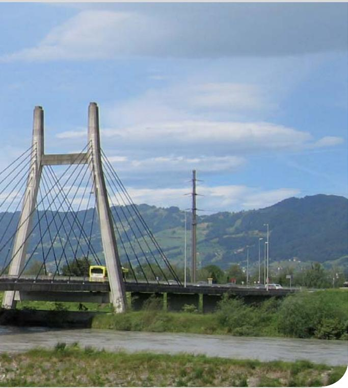
cialists are expecting to be able to measure substantial movements there, above all due to the effects of wind and temperature fluctuations. A Leica TM30 total station and prisms will be installed at a later date.
