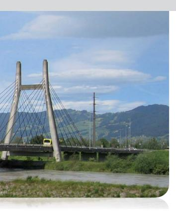
cialists are expecting to be able to measure substantial movements there, above all due to the effects of wind and temperature fluctuations. A Leica TM30 total station and prisms will be installed at a later date.
