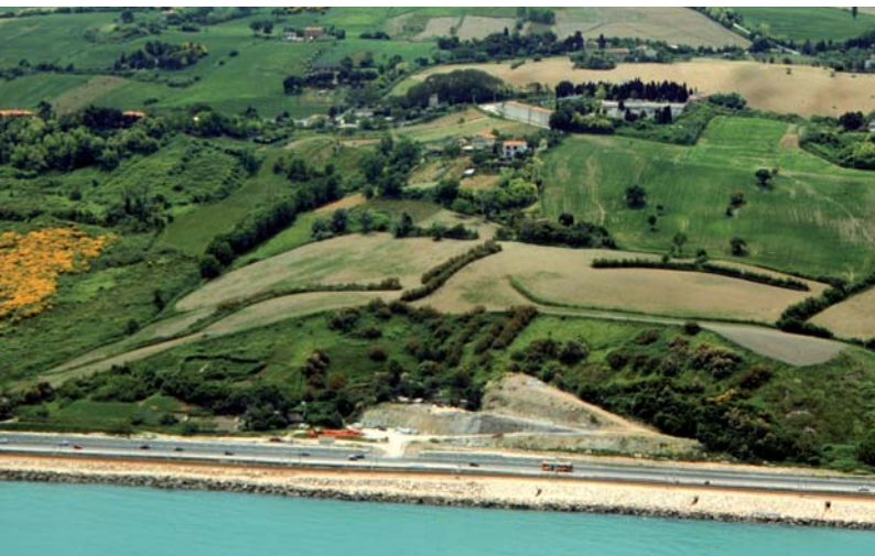
■ View of the "Great Ancona Landslide" today.
