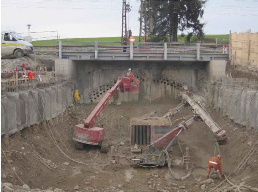
Installation of pipe canopy tunnel lining (monitoring phase II)
