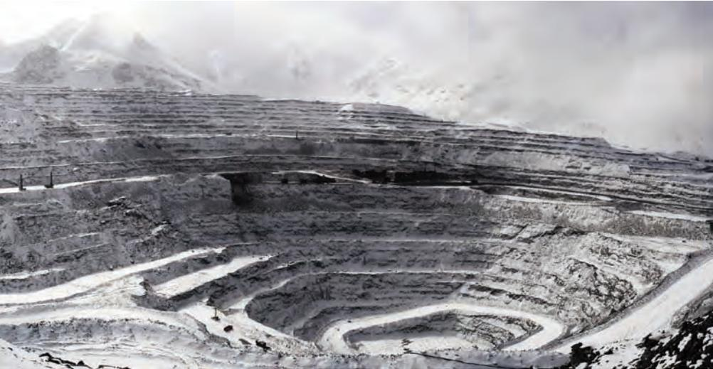
**Since 2003 the Kumtor gold mine has been using Leica GeoMoS as their main automatic deformation monitoring system. Periodic manual monitoring and geotechnical instrumentation are still in use for added safety.**
