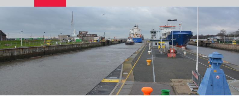
lock gate at 14m below sea level. The chamber will be built into the sluice island between the large and small locks and requires the removal of roughly 1.6 million m<sup>3</sup> of mostly clay soil. Three months of monitoring the existing lock system at Brunsbüttel was necessary in order to analyse the stability of the structure before starting with construction. Once the project began, the seven-year construction site will be monitored until its completion.
