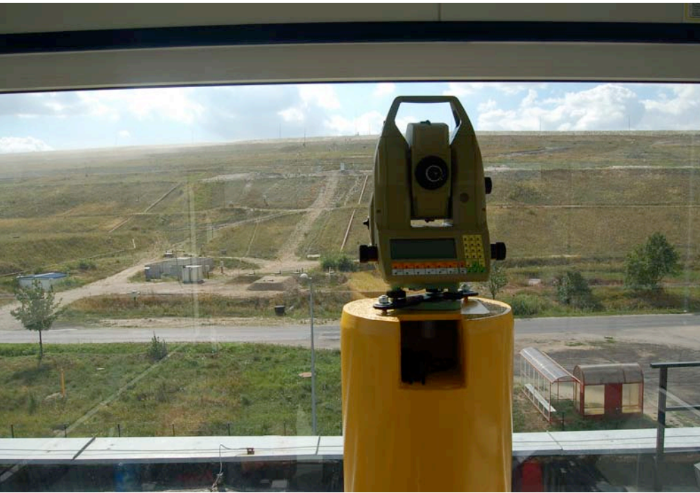
View from the monitoring hut towards the tailings dam wall.
