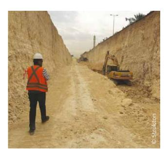
Strukton, in charge of Line 6 (Purple), has been tasked with capturing data for topographic surveys, as-built checks, volume calculation, and inventory of existing utilities. The technology company specialising in rail systems and civil infrastructure is also in charge of stakeouts for construction and deviation monitoring.
