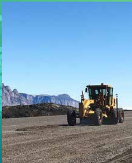
Runway maintenance with machine control in Greenland
