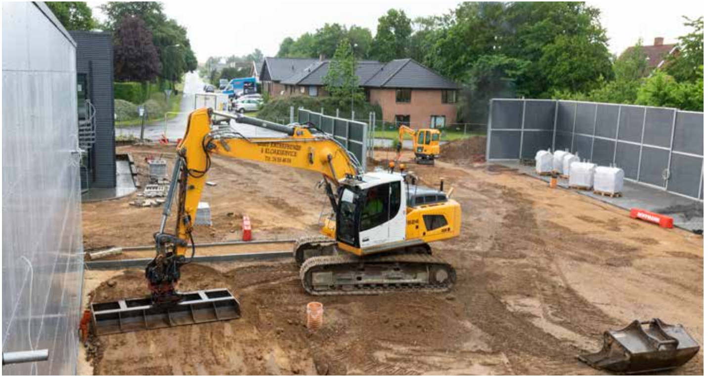
The Liebherr 924 working with Leica iXE3, rototilt and a grading beam.
