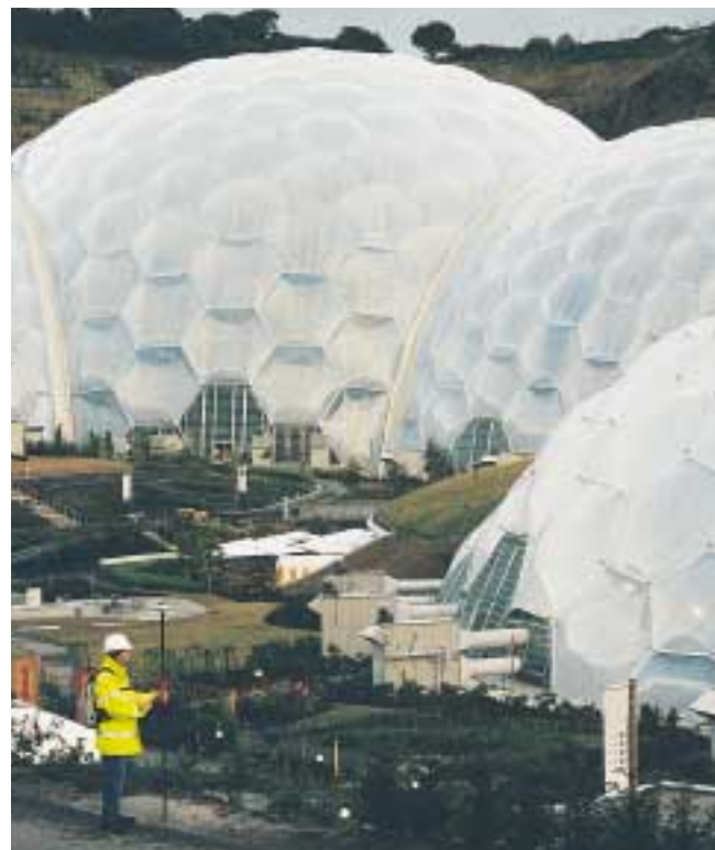
Above: Tim Hall, from Ordnance Survey measures at the Eden Project – an immense greenhouse landscape under geometrical domes. He uses a Leica GPS with RTK corrections delivered by GSM phone link from his Truro office some 27 kilometres away to revise 1:2500 mapping.
