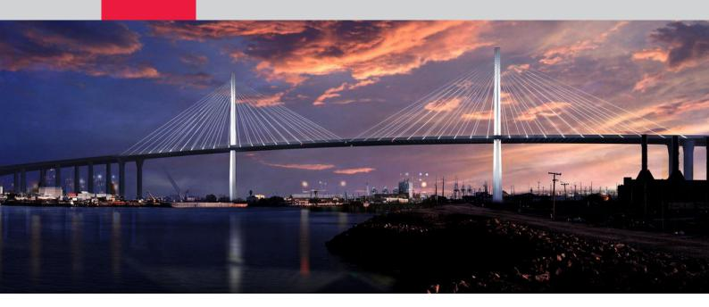
of Structural Monitoring David Rutledge. "As the structure began to climb in height, maintaining line of sight to the prism would become increasingly difficult. The Leica solution is to gracefully switch over to the GNSS system for primary alignment control. This is a proven methodology that has been used on the world's largest buildings."
